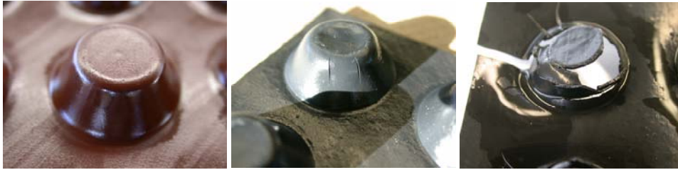
(a) No failure (b) Cracking (c) Severe cracking
